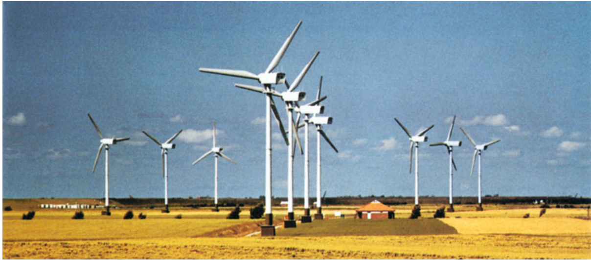
Figure 8.49 Windfarm Krummhörn. Rotor span width is 30 m, the nominal electric power output is 300 kW per wind converter. (With kind permission of EWE corporation, Oldenbourg)
