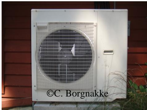
The compressor is inside the unit to the left that also houses a fan and the heat exchanger.
