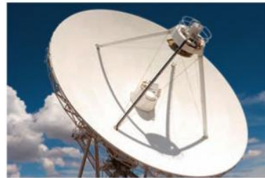
Dish antennas are paraboloids of revolution
