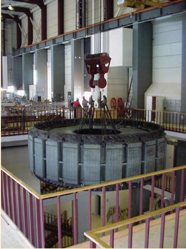
■ FIGURE 12.21 The 24-pole rotor of a synchronous generator as it is being lowered into position.
