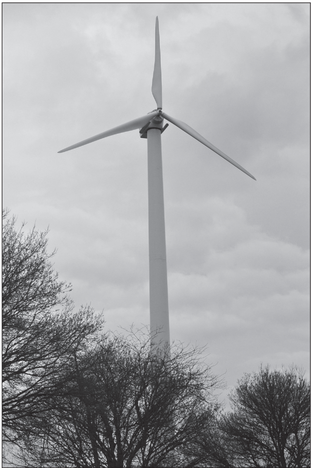
Wind turbines will play a large role in our energy future. The photo shows a 100 kW HAWT, installed in 2011 at the Fisherman’s Memorial State Camp Ground in Narragansett, Rhode Island. It is programmed to generate 100 kW in winds from 13 to 25 m/s and supplies half the electricity needed for the camp’s 18,000 annual visitors. Wind energy is good, but expensive. This turbine cost more, just to install, than it will recover in power savings over its 20-year life span. [Dr. Frank M. White]
