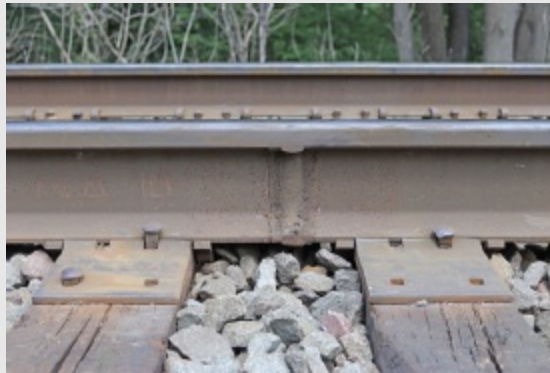
CS Photo 9.2 Track using continuous welded rail, showing one of the welded joints.
