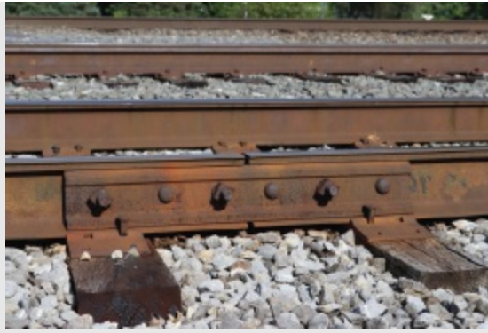
CS Photo 9.1 Track with bolted joint bars connecting the rails.
