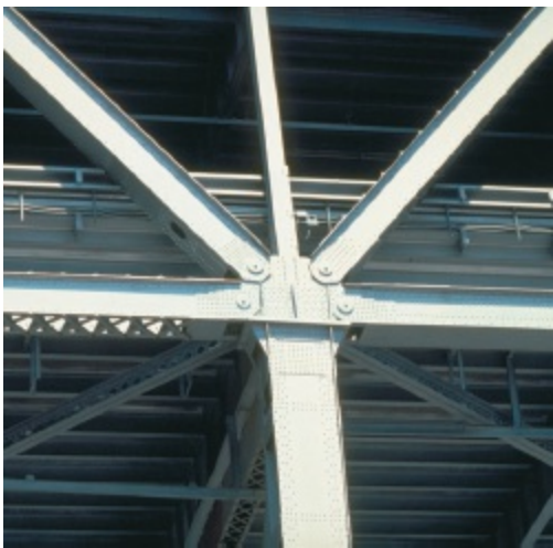
Photo 6.2 Shown is a pin-jointed connection on the former approach span to the San Francisco–Oakland Bay Bridge.
