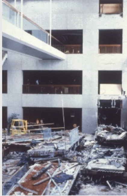
CS Photo 2.1 Wreckage of walkway collapse. Note that the third-floor walkway remained intact.
