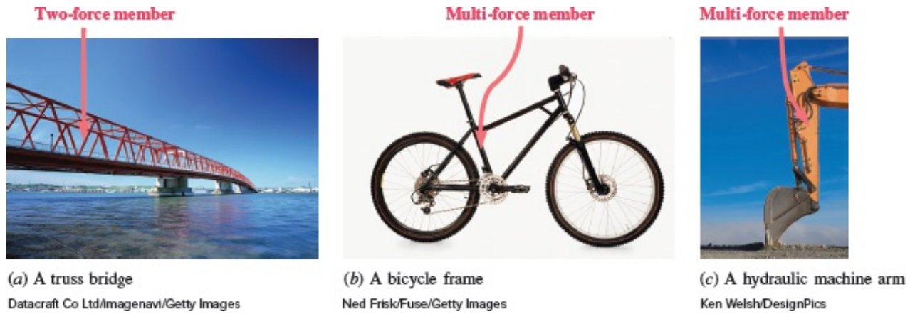
Photo 6.1 The structures you see around you to support loads or transmit forces are generally trusses, frames, or machines.
