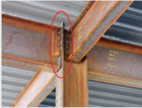
CS Photo 4.1 Bolted double-angle simple shear connection (circled). Courtesy of AISC
