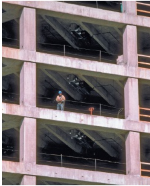
Photo 11.4 Reinforced concrete building frame.
