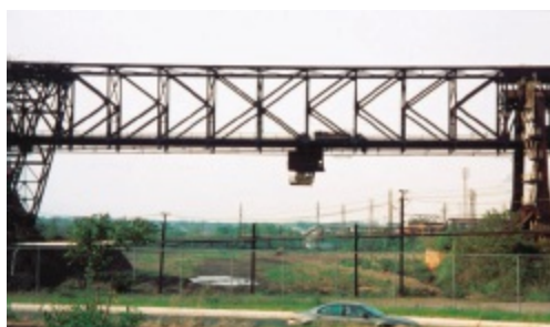
Photo 6.3 Two K trusses were used as the main components of the movable bridge shown, which moved above a large stockpile of ore. The bucket below the trusses picked up ore and redeposited it until the ore was thoroughly mixed. The ore was then sent to the mill for processing into steel.
