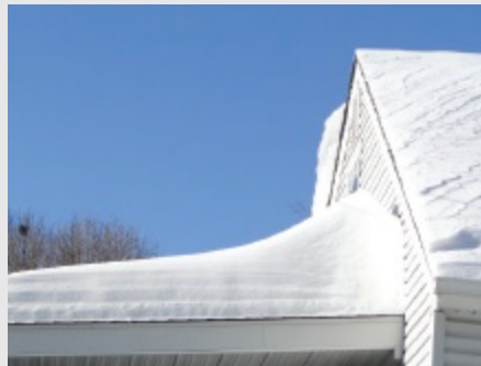
CS Photo 5.1 Drifting snow on a lower roof, with depth increasing toward the upper structure.
