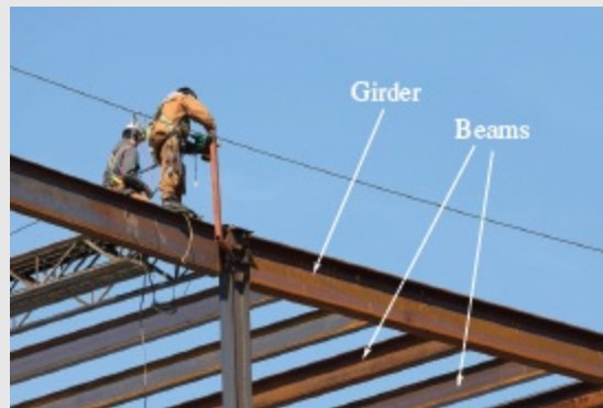
CS Photo 15.2 View of floor framing (prior to placement of concrete deck).
