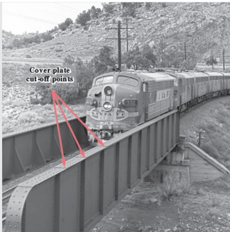
CS Photo 7.1 Riveted through plate girder bridge.
