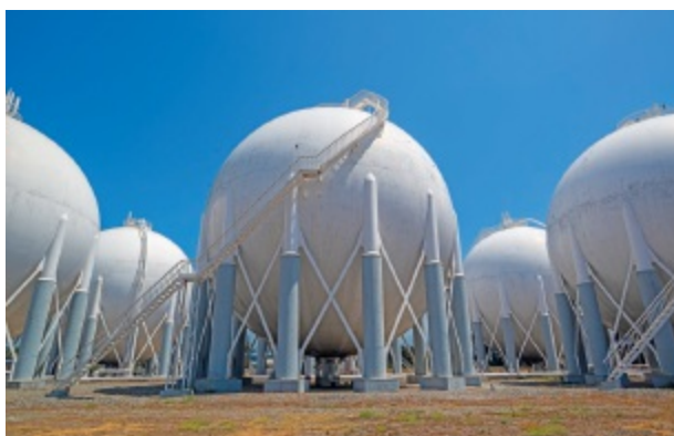
Photo 14.4 Spherical pressure vessels at a chemical plant.
