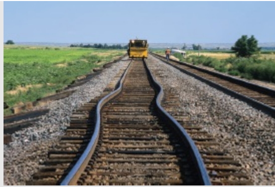
CS Photo 9.4 Track that buckled due to elevated ambient temperature conditions.
