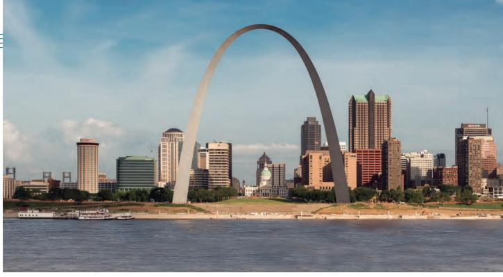
The Gateway Arch in St. Louis, Missouri, stands 192 meters high and was completed in 1965. The arch was designed by the architect Eero Saarinen using an equation involving the hyperbolic cosine function. In Exercise 8.1.50 you are asked to compute the length of the curve that he used.
