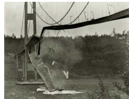
FIGURE 5.R.6 Collapse of the Tacoma Narrows Suspension Bridge
