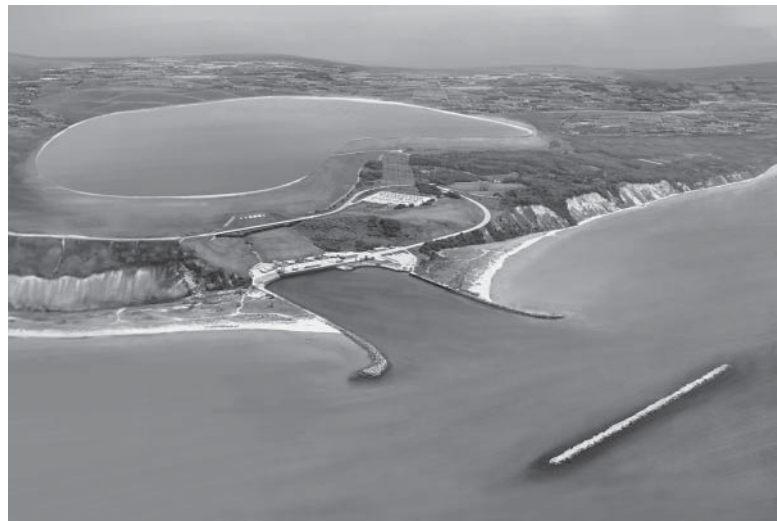
FIGURE 3.34 The world's largest artificial hydro-storage facility in Ludington, Michigan, pumps water 100 m above Lake Michigan when excess power is available. It can deliver 1800 MW when needed from reversible pumps/turbines.
