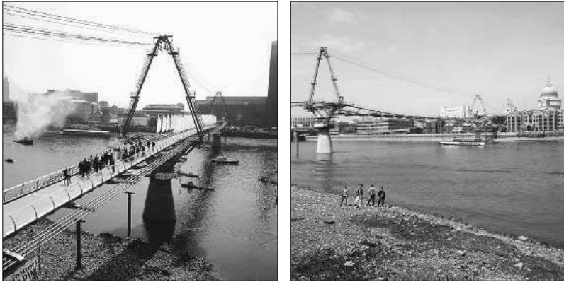
FIGURE 4.28 Millennium Footbridge, London. (Courtesy of Ove Arup & Partners, Engineers.)
