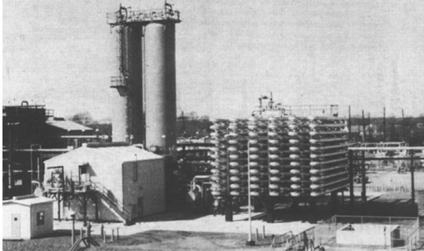
Figure 2-9 Dimersol G (an organometallic catalyst) unit (two CSTRs and one tubular reactor in series) to dimerize propylene into isohexanes. Institut Français du Pétrole process. Photo courtesy of Editions Technip (Institut Français du Pétrole).
