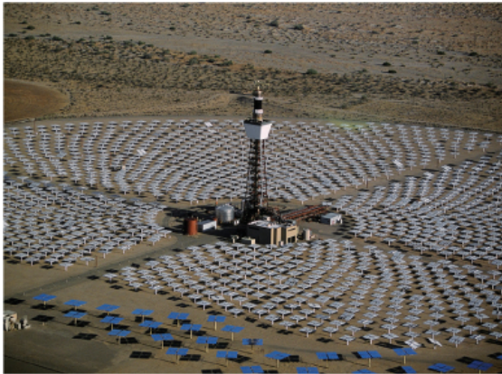
Figure P8-16 B Solar field design. Five 265-m-tall towers with three heliostat fields/tower, on 275 acres of land in Daggett, CA. Net concentration 3,868 suns and 295 MW delivered to each solar reactor. (Melinda M. Channel, Jonathan Scheffe, Allan Lewandowski, and Alan W. Weimer, November 11,
