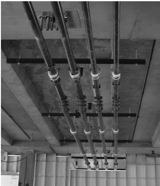
FIGURE 21.3 Mechanical equipment post-installed in a concrete slab. (Photograph by Charles W. Dolan.)
