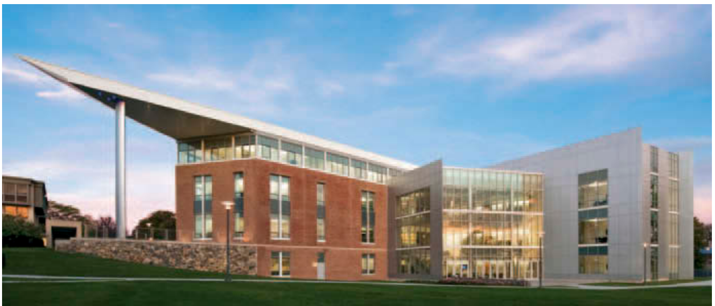
Figure 4.19 The bay-side elevation as built. Note metal-clad “fin walls” express the radiating geometry (© Anton Grassl/Esto).
