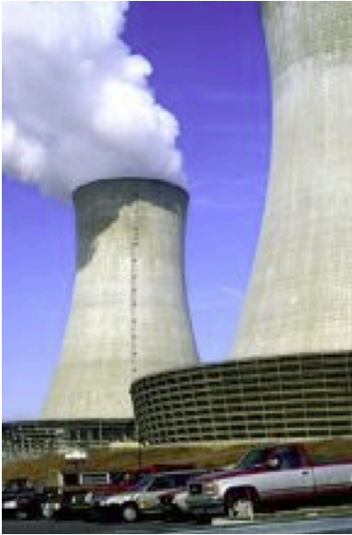
Figure 8.9 Natural-draft cooling towers in a nuclear power plant. The packing occupies only the bottom section; the rest of the tower acts as a chimney to create the flow of air (Courtesy of Michael Rennhack, Nuke-Worker.com).
