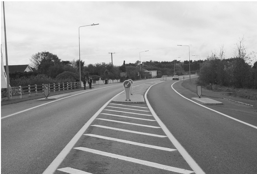
Figure 11.2 Speed control by road narrowing.
