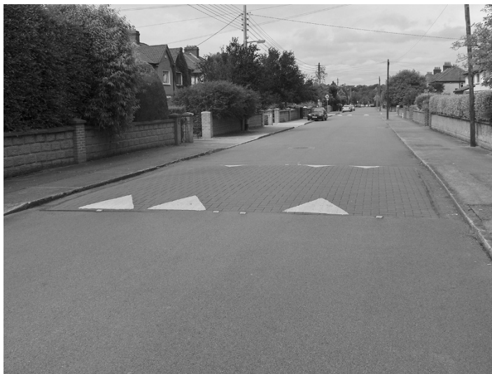
Figure 11.1 Speed control by the installation of a traffic ramp.
