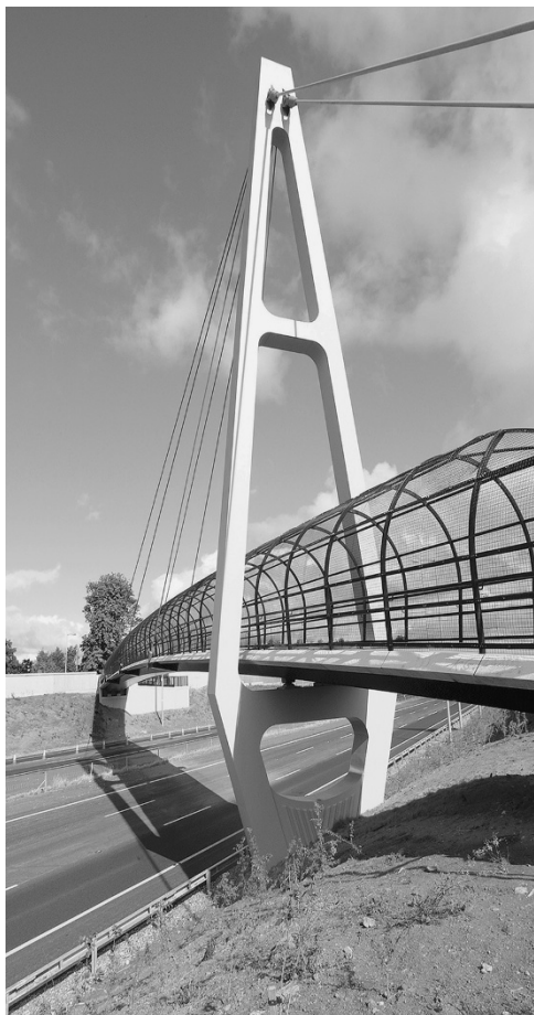
Figure 3.3 Footbridges can lessen effects of severance.
