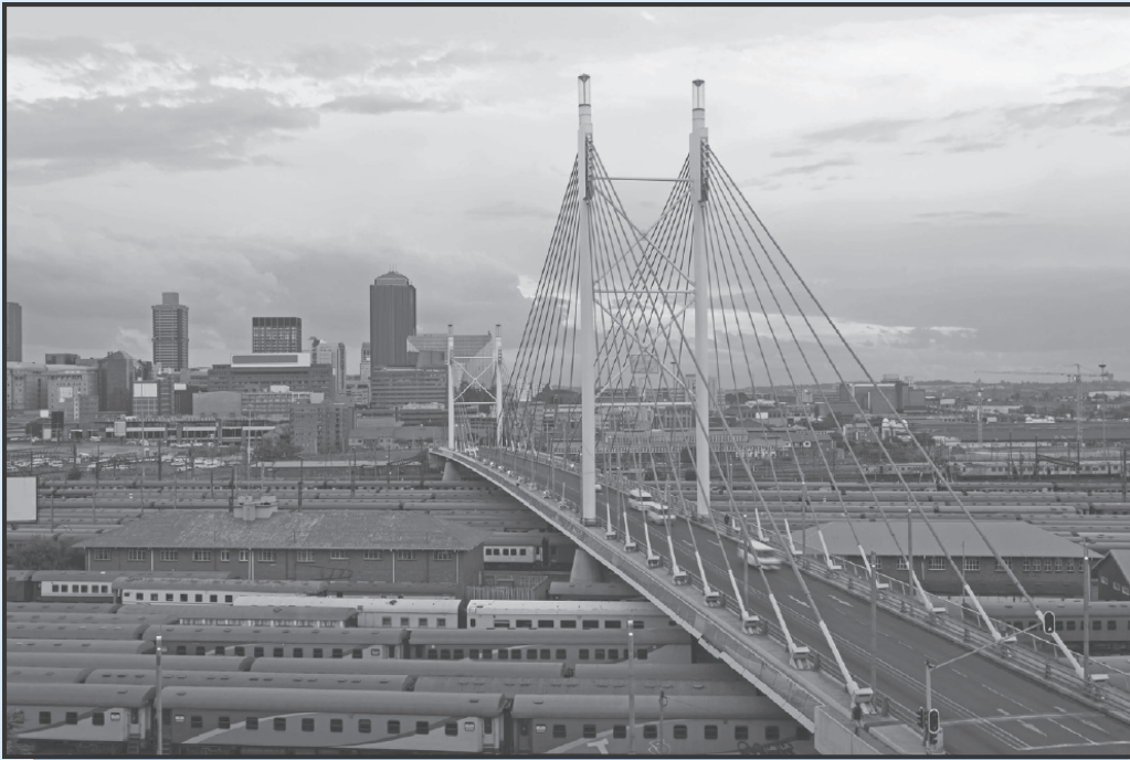
Figure 11.10 Nelson Mandela Bridge, Johannesburg.
