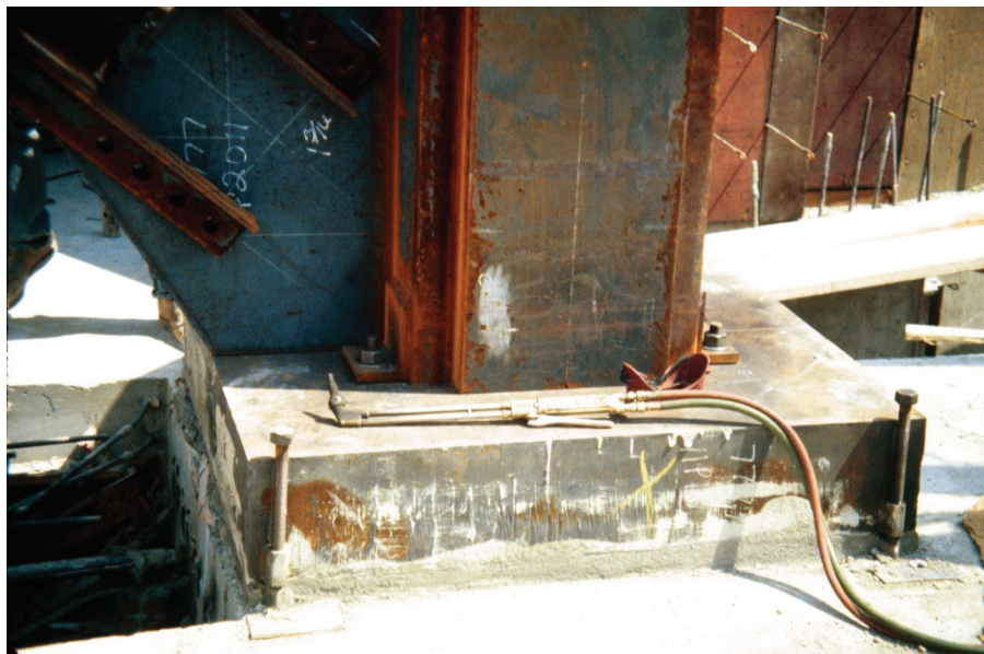
Fig. 4-16. Base plate with adjusting screws.
