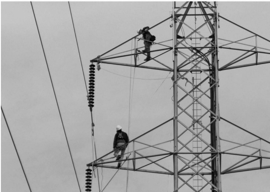
FIGURE 1.4 A transmission line is being upgraded.
