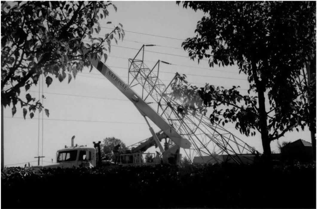
FIGURE 1.3 Installation of a 345 kV double-circuit transmission tower made of a steel cage.
