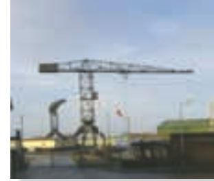
Simple trusses are often used in the construction of large cranes in order to reduce the weight of the boom and tower. (© Russell C. Hibbeler)
