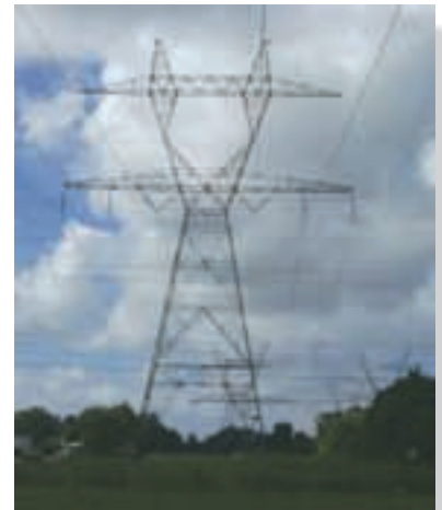
For economic reasons, large electrical transmission towers are often constructed using space trusses. (© Russell C. Hibbeler)
