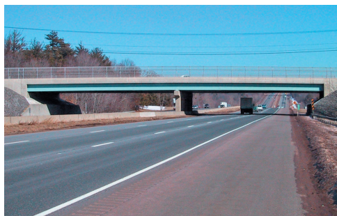
Photo 15.2 The continuous beams supporting this highway overpass have three supports and are thus statically indeterminate.
