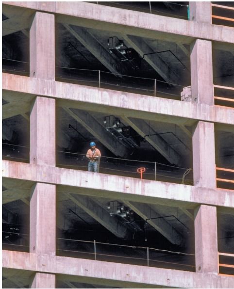
Photo 11.4 Reinforced concrete building frame.
