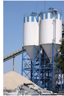
Photo 5.3 The storage tanks shown are bodies of revolution. Thus, their surface areas and volumes can be determined using the theorems of Pappus-Guldinus.
