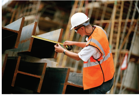
Photo 7.1 Appendix B tabulates data for a small sample of the rolled-steel shapes that are readily available. Shown above are examples of wide-flange shapes that are commonly used in the construction of buildings.
