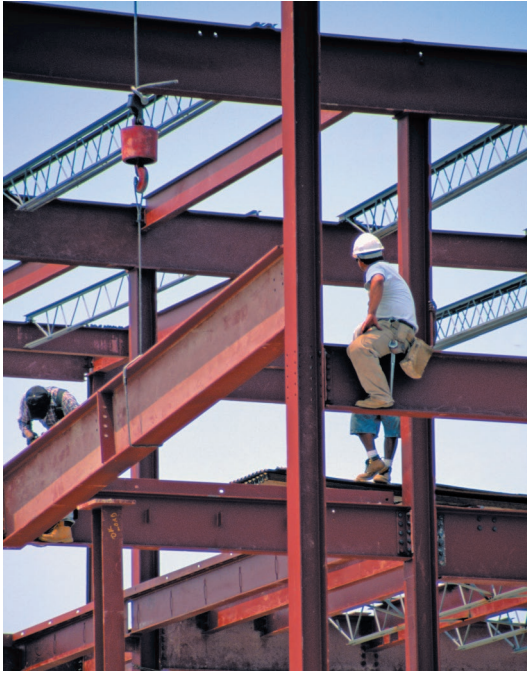
Photo 11.3 Wide-flange steel beams are used in the frame of this building.
