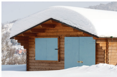
Photo 5.4 The roof of the building shown must be able to support not only the total weight of the snow but also the nonsymmetric distributed loads resulting from drifting of the snow.
