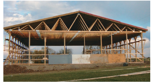
Photo 6.4 Because roof trusses, such as those shown, require support only at their ends, it is possible to construct buildings with large, unobstructed interiors.
