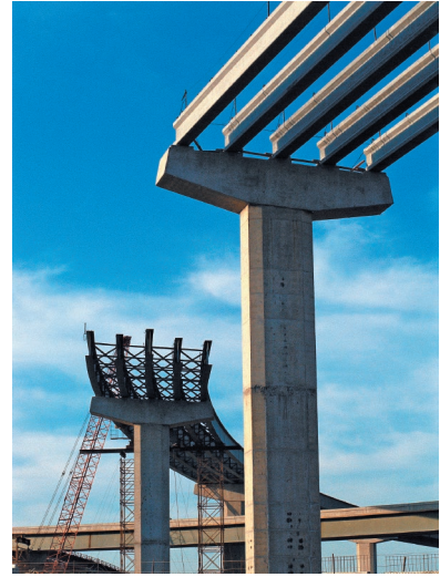
Photo 15.1 A different function M(x) would be required in each portion of the beams when a vehicle crosses the completed bridge.
