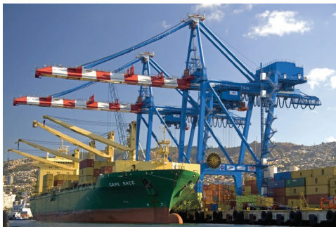
Photo 8.3 Crane booms used to load and unload ships.
