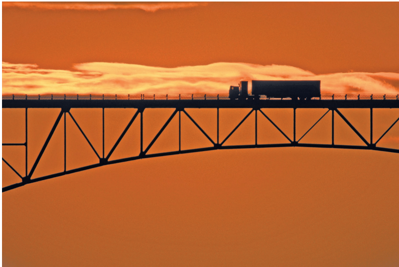
Photo 8.1 This bridge truss consists of two-force members that may be in tension or in compression.
