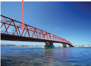
(a) A truss bridge
