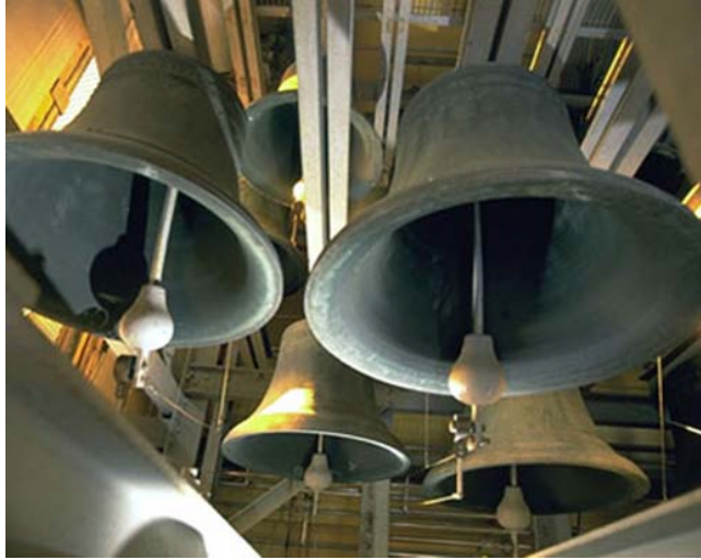
Figure 5.1.1 A vibrating system with very low and very high natural frequencies. Wallace Memorial Carillon. Reproduced by permission from Christ Church Cranbrook
